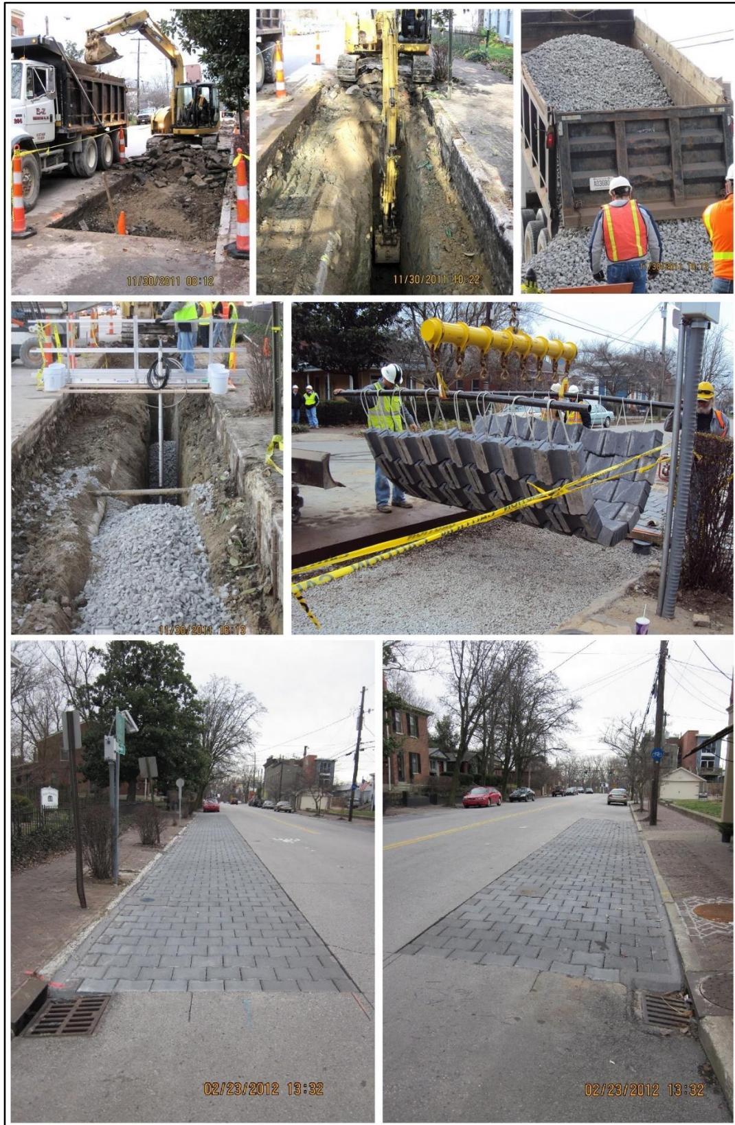
Figure 13 - Construction Stages of Controls 19G & 19H
