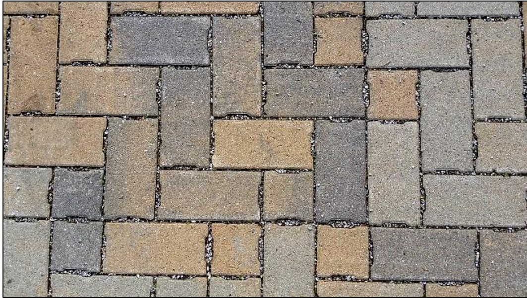
Figure 7 - An Application of Permeable Interlocking Concrete Paver in Louisville, KY
