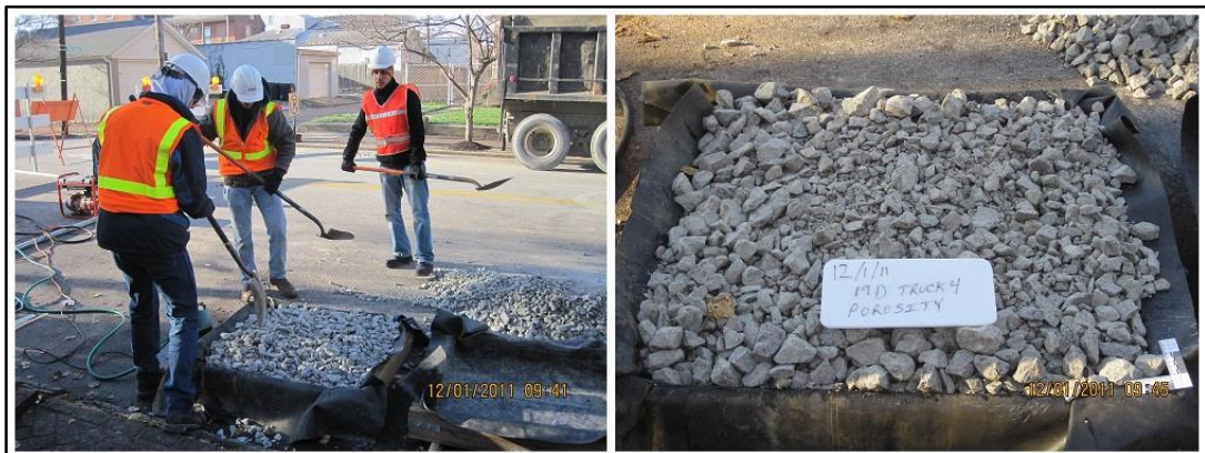
Figure 21 - Porosity Measurements during Construction of Controls 19G & 19H
